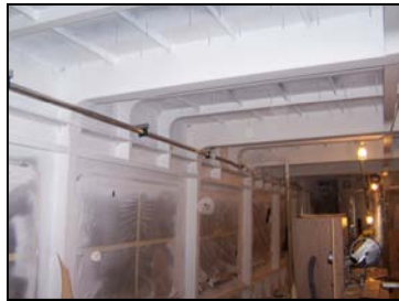
Typical spray application
