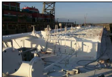
View of a barge after application
